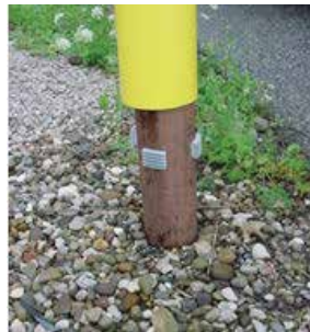
Step 2 - Place cover over grip tabs.
