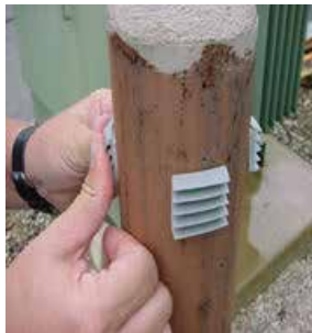
Step 1 - Install self-adhesive grip tabs.
