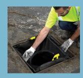
2. Place the filter into recess and adjust the wire frame to fit the outside edges
