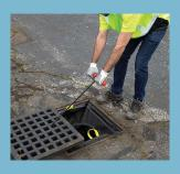
3. Once the insert is properly positioned on the lip of the catch basin, reinstall the grate.
