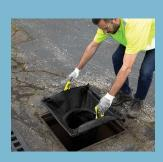
**TO REMOVE:** Simply remove grate and lift the Storm Sentinel® out by the handles.
